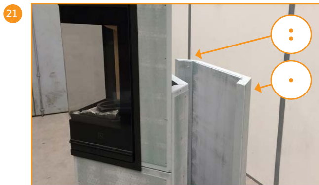
Glue the three upper rear pieces together with the side pieces and fasten with three screws
