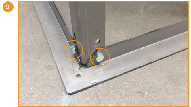
Important! When mounting the surround plates, the rear side must fit closely against the head of the bolt
