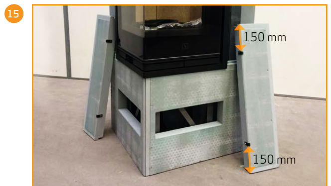
Mount the side pieces with two fittings. NOTE: These do not have a hole pattern
