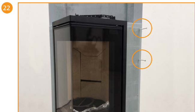
Glue the side pieces to the rear piece and fasten with two screws
