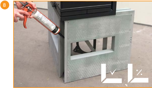
Push the front pieces together and glue them so that the bevels fit together
